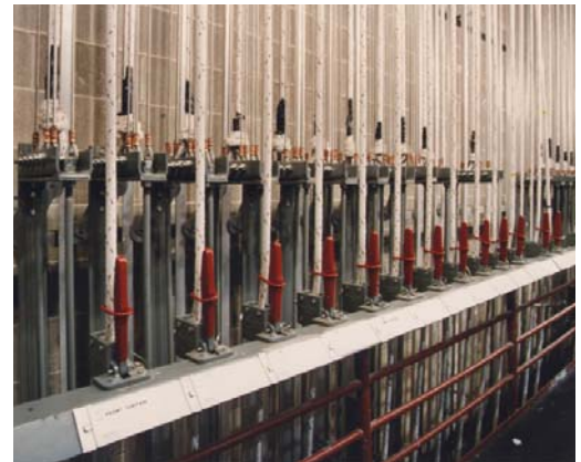
Typical Underhung Counterweight System
